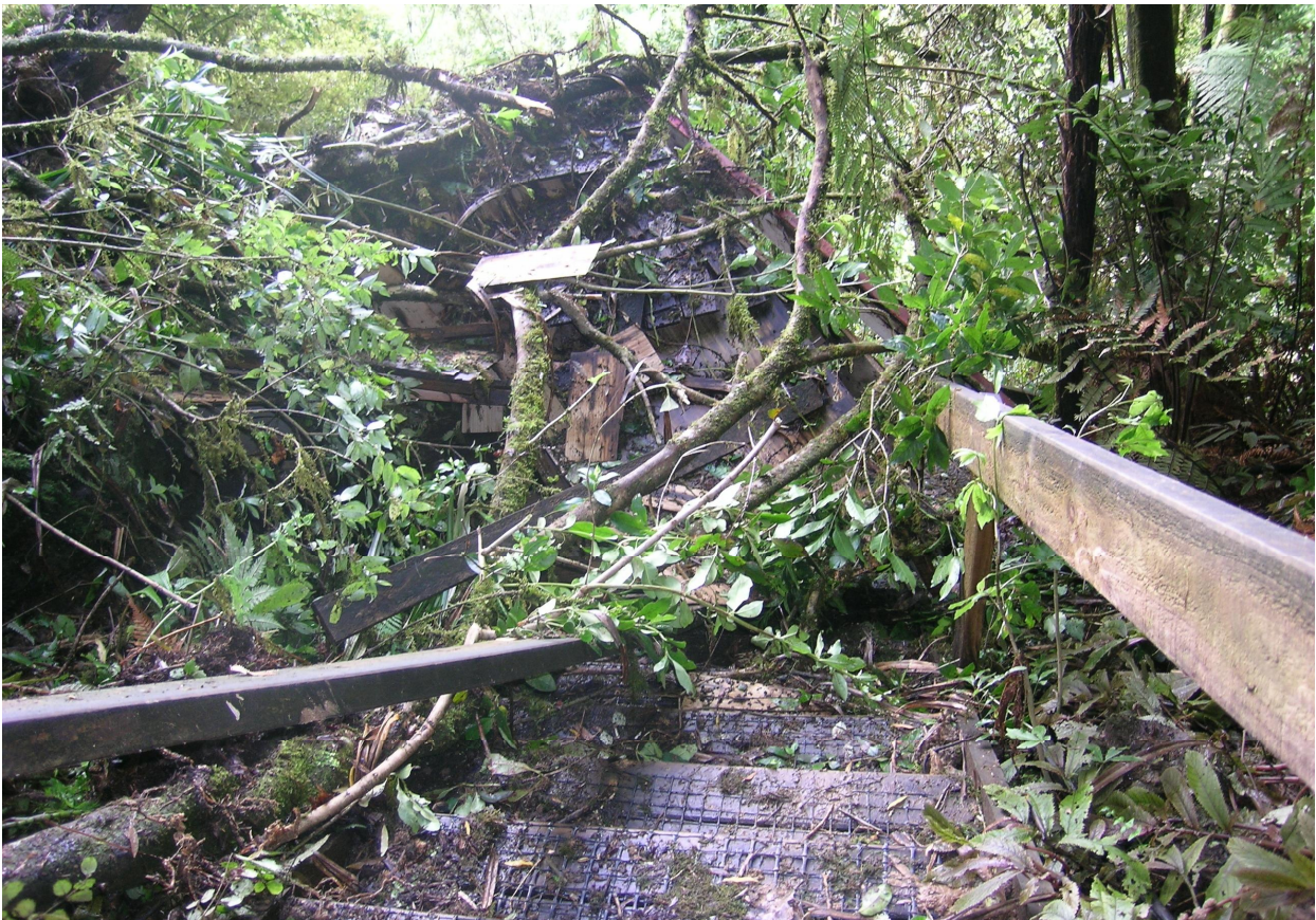
The demolished Visitor Shelter at Aranui Cave. Photo: Dave Smith.
